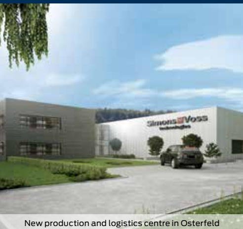
New production and logistics centre in Osterfeld
